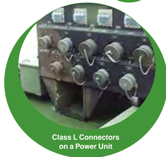
Class L Plug and Receptacle
